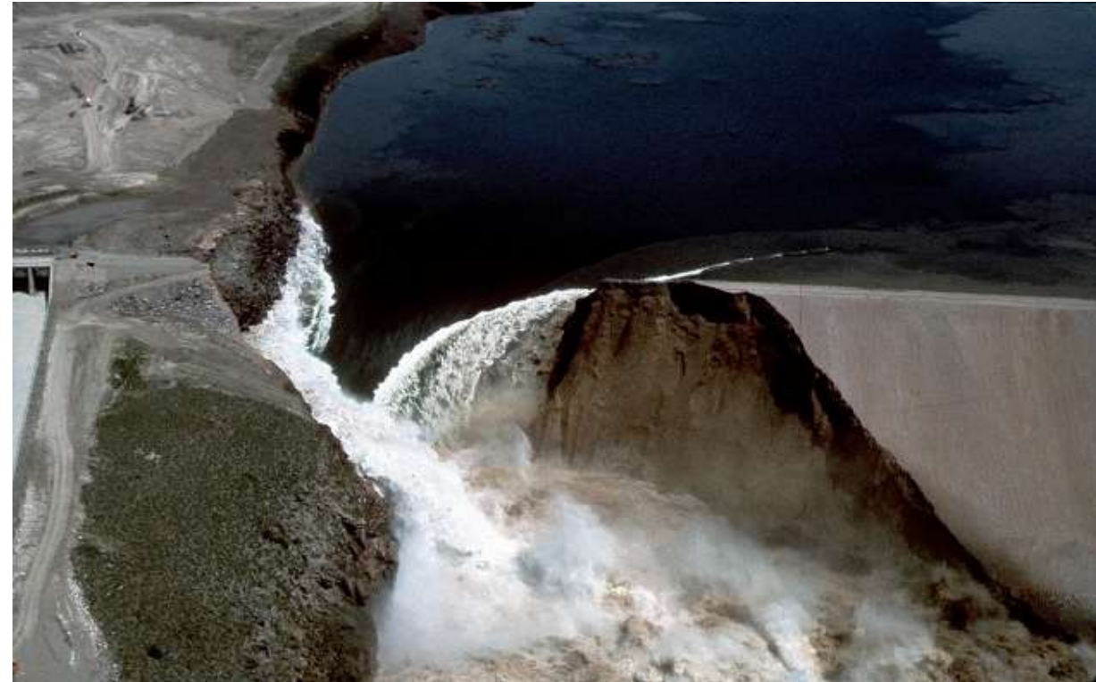
View of the dam breach early afternoon
