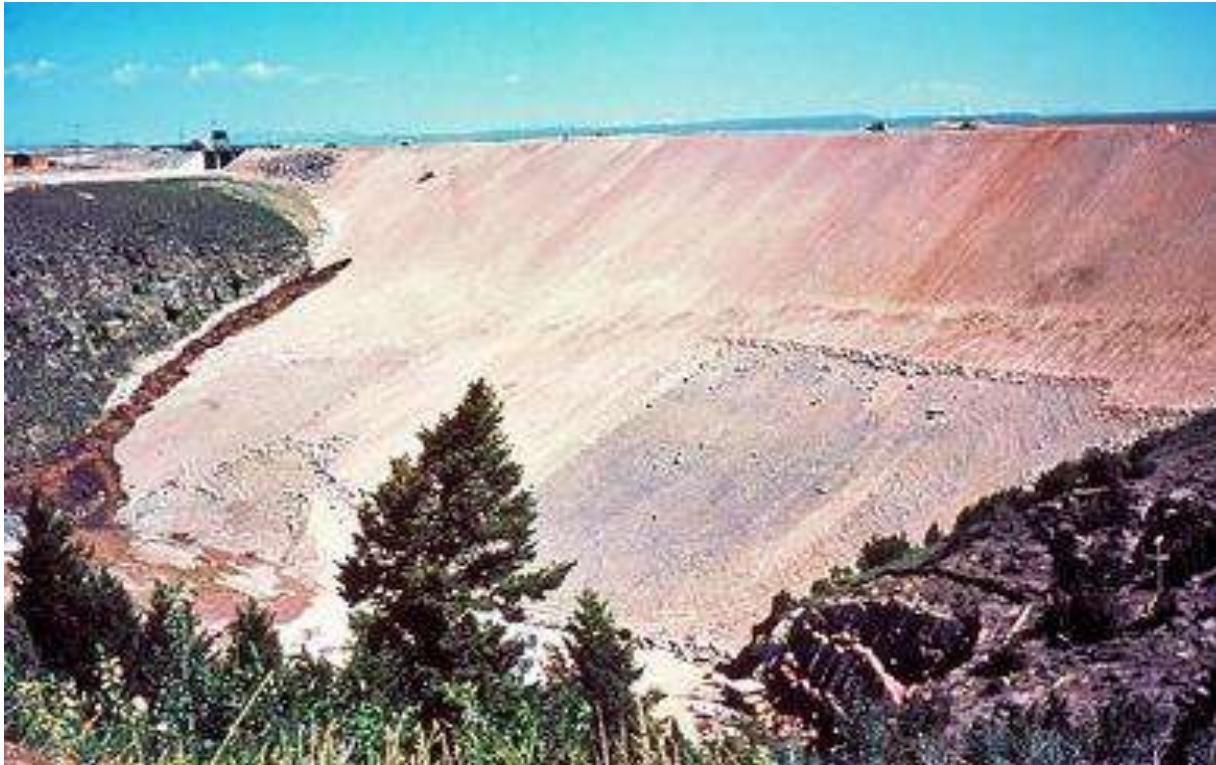
View of the spring on the right abutment at 10:30
