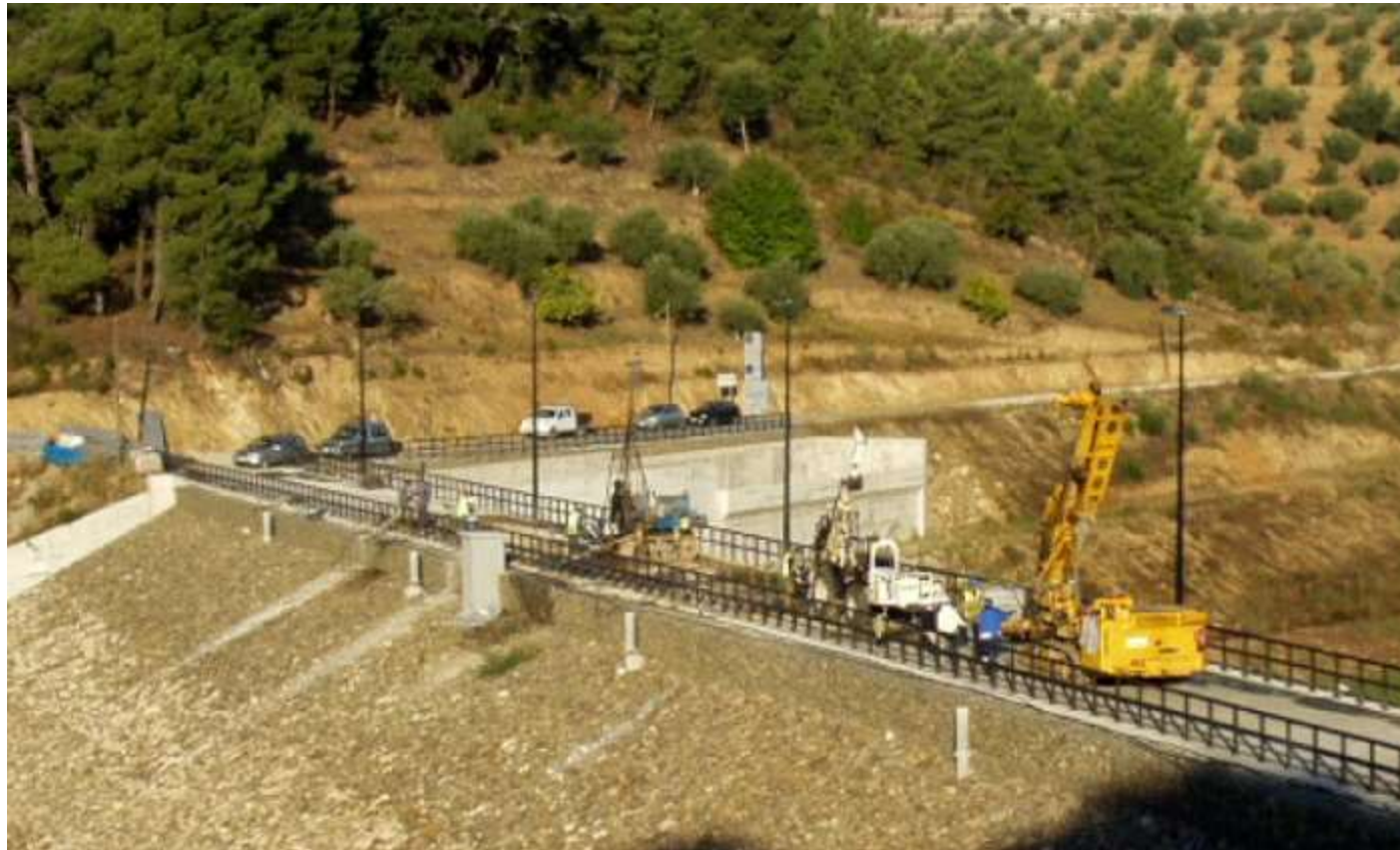
Execution of the grouting curtain from the dam crest
