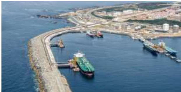
LIQUID BULK TERMINAL
