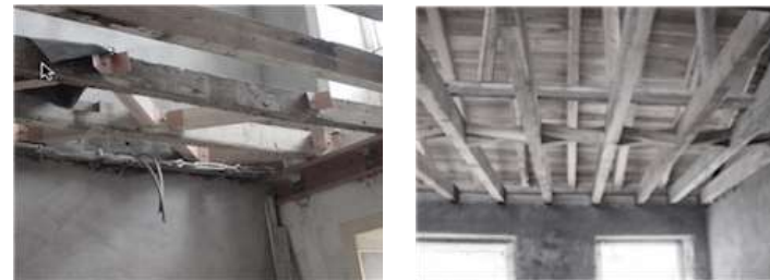
FLOOR STIFFENING WITH DIAGONAL BRACING AND TIMBER PLANKS
