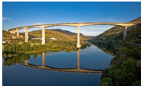
Fig. 8: Ponte Miguel Torga – Portugal (1997)
