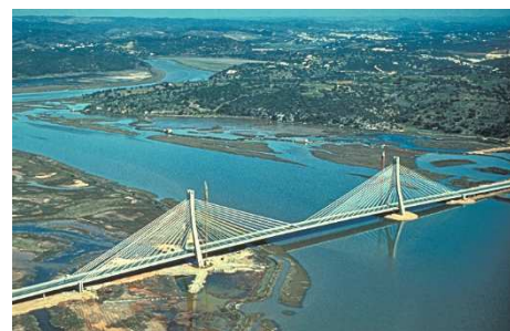
Fig. 14: Ponte do Arade – Portugal (1991)
